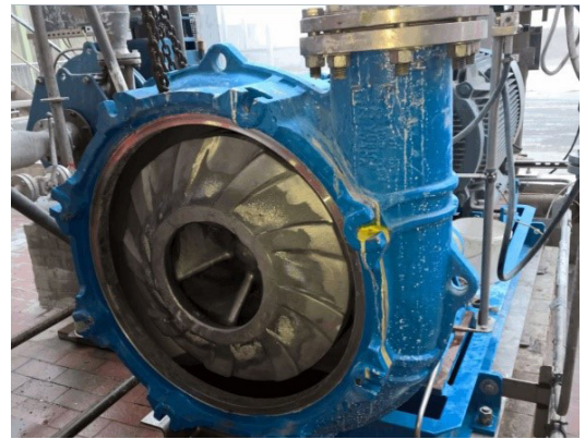
EMW pump during inspection
